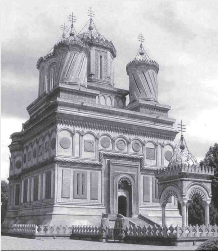
FIGURE 1. The Monastery of Arges as it appears in modern times. Photograph by Ruxandra Ion.
